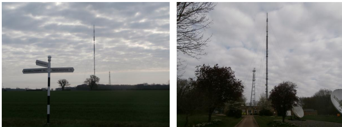
Figure 14 The “new look” of Tacolneston after work was completed to remove the old tower.
