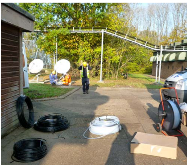
Figure 3: The three measured air sampling lines coiled up on the day of installation with the riggers in the background preparing the proprietary cleats for attaching the tubing at 1 m intervals (left). The right hand image shows the new tall tower at Tacolneston on the left, where our sample lines are installed, with the obsolete historic tower in the centre and the smaller but still operational tower on the far right.
