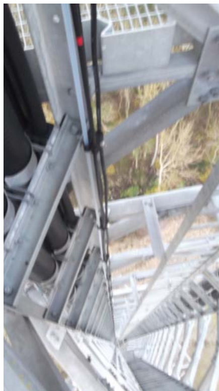
Figure 2: The 100 meter line installed in the tower at Tacolneston. The attachment of the air sampling line to the stainless steel cup is shown on the left and two of the air sampling lines running down through cleats is shown on the right.
