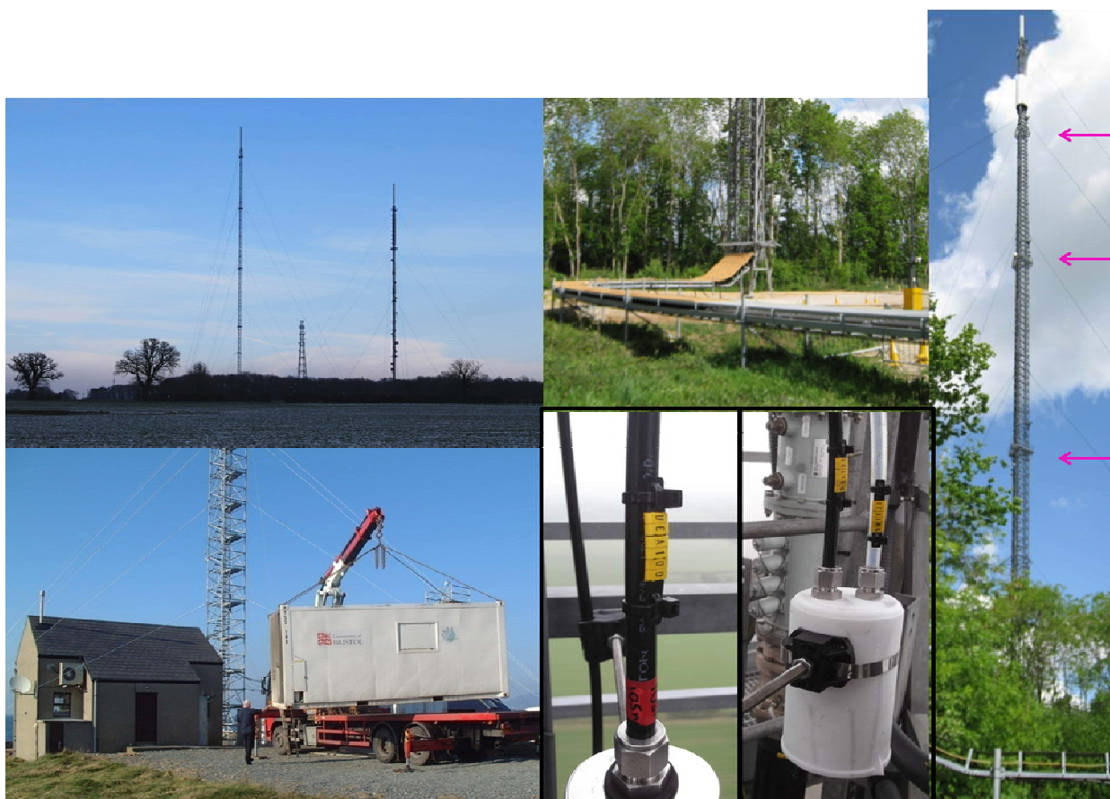
Figure 4: The approximate location of the air sampling lines (180 m, 100 m, 50 m) on the tower at Tacolneston (right). The cups which cover the line inlets at the top of the tower (lower centre) and the mobile lab (bottom left) which will house instrumentation at Tacolneston.
