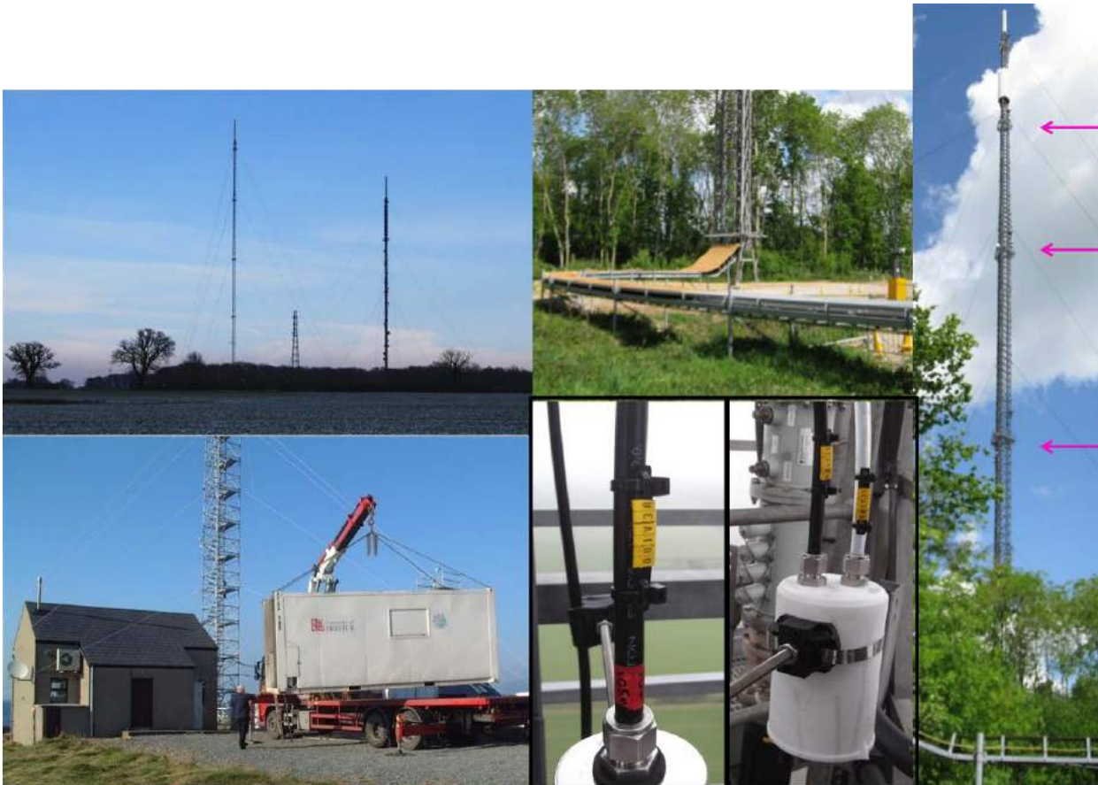
Figure 158: The approximate location of the air sampling lines (185 m, 100 m, 54 m) on the tower at Tacolneston (right). The cups which cover the line inlets at the top of the tower (lower centre) and the mobile lab (bottom left) which will house instrumentation at Tacolneston.
