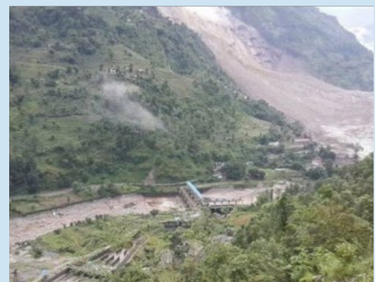
The Sunkoshi Hydropower station was damaged by the rain-triggered landslides in 2014.
