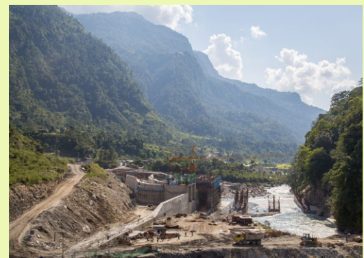
Construction of the Upper Marsyangdi Hydroelectric Station.
